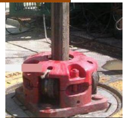
Drill floor with Rotary Table, Kelly and Kelly bushing
